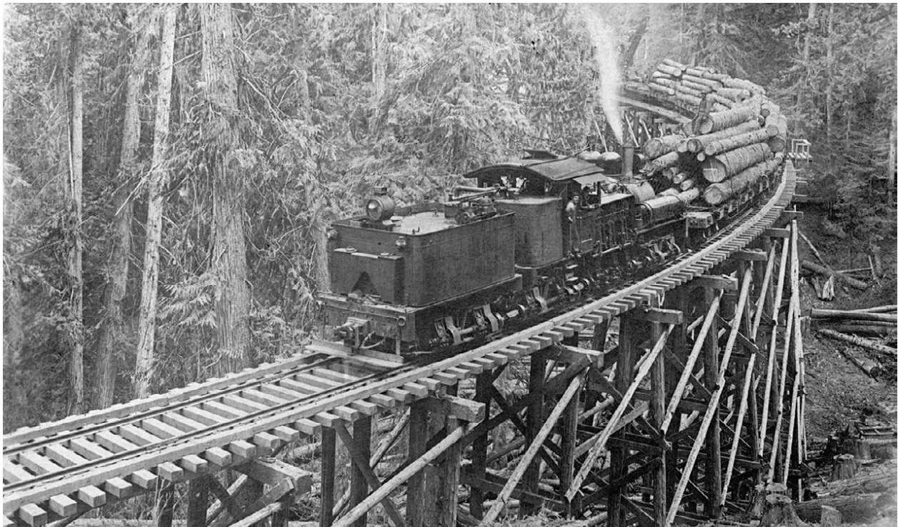
ABOVE: Logging railroads all across the Mountain West were built inexpensively and with the materials at hand. This massive curved timber trestle on Idaho's Blackwell Lumber Company railroad holds a three-truck Shay and its log train in this 1910 postcard.
